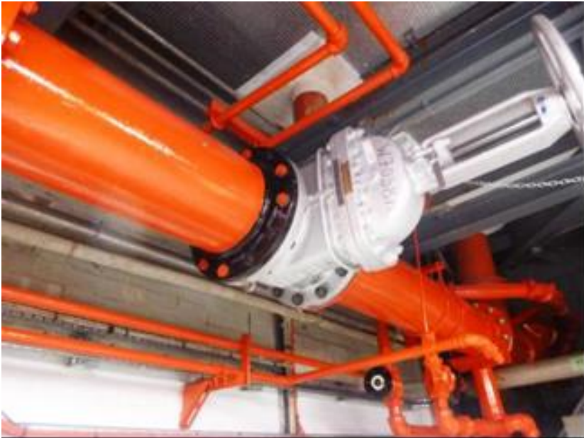
Completed remediation on gas circulator fire pipework
