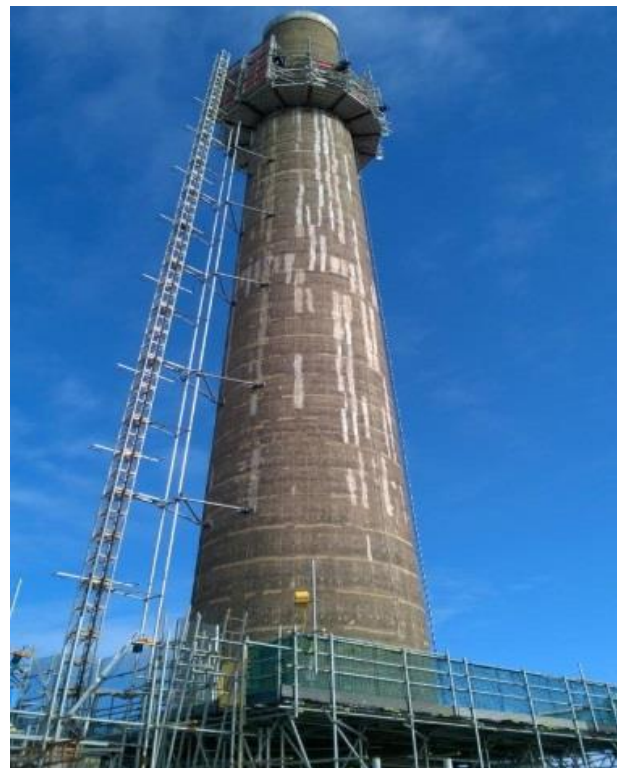
First Generation Magnox Reprocessing Plant stack – height reduced 2017-18
