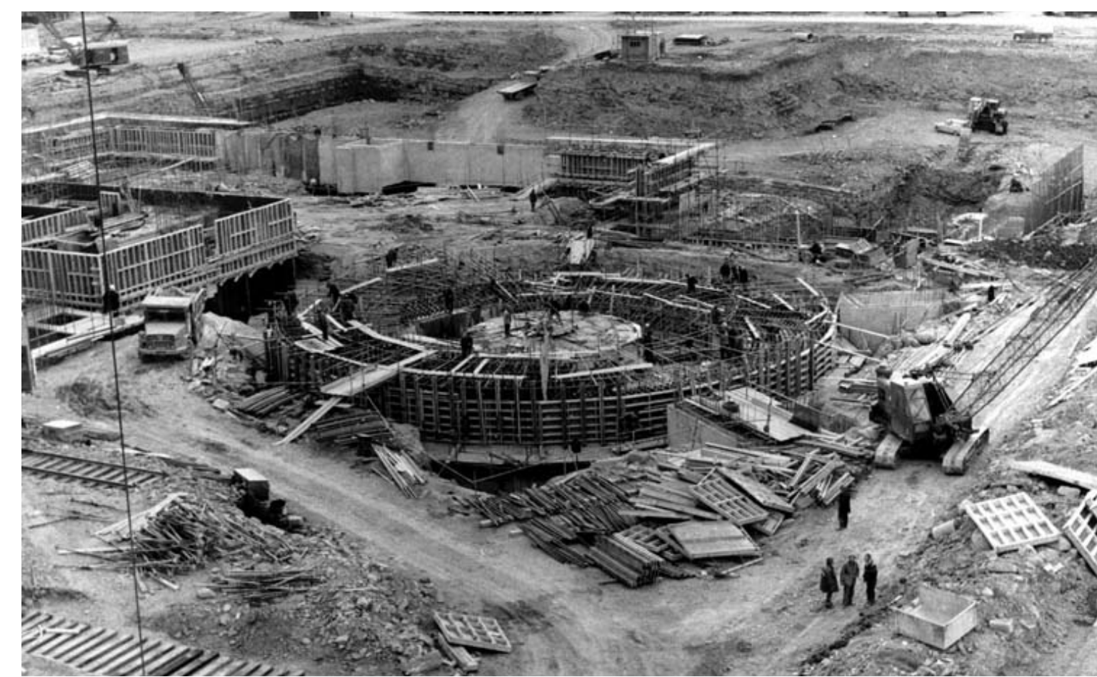
Reactor 4 at Hinkley Point B under construction
