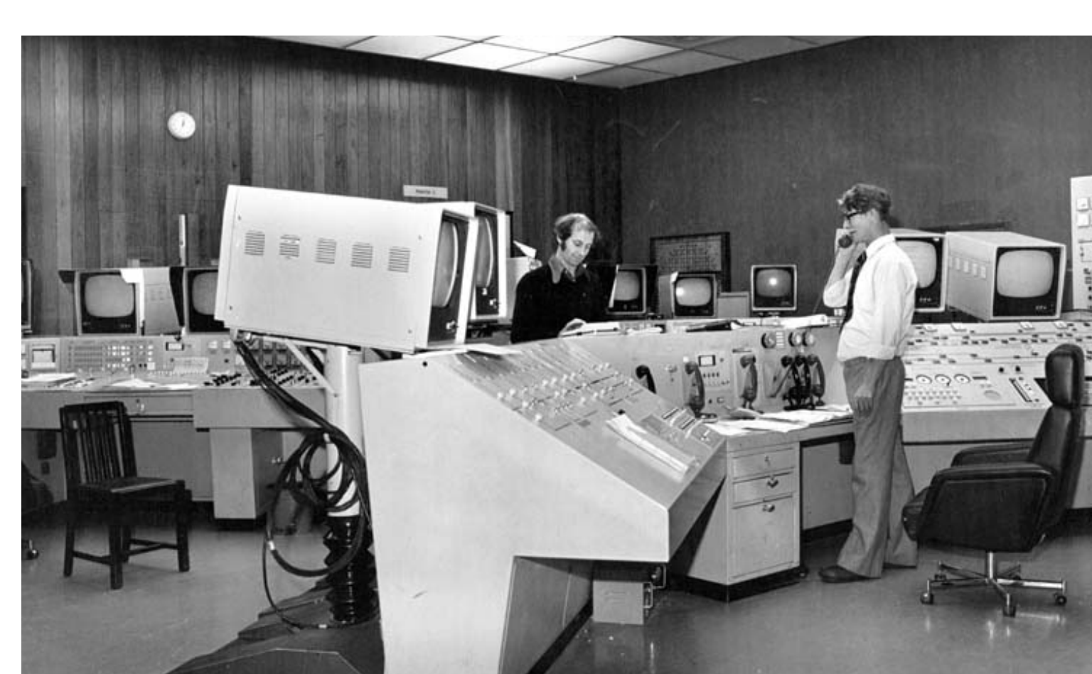
Hinkley Point B main control room
