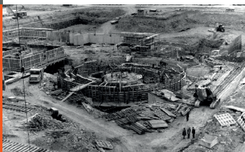
Reactor 4 at Hinkley Point B under construction
