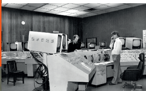
Hinkley Point B main control room
