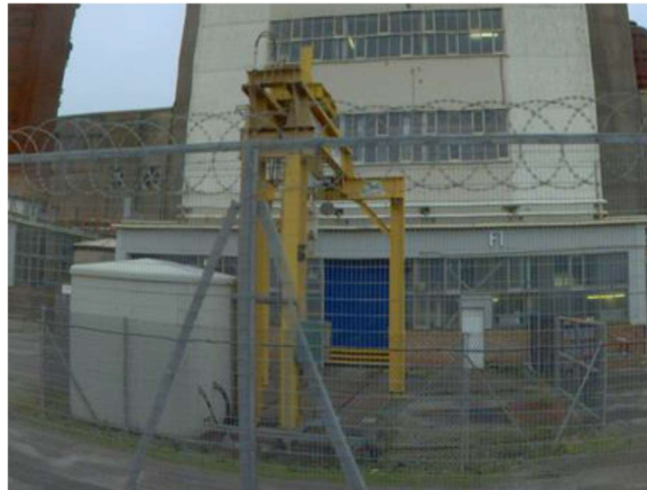
Figure 4: Reactor 1 Gallows hoist before removal.
