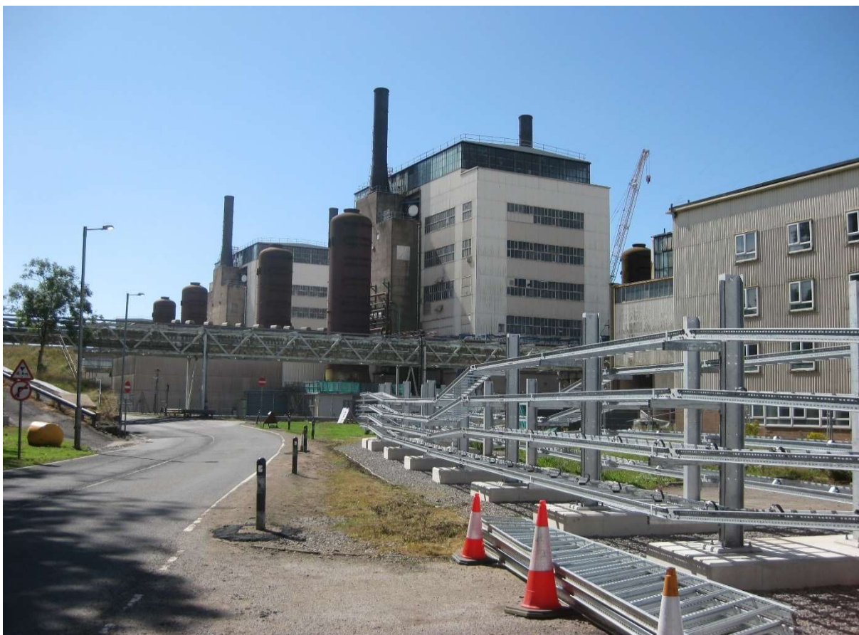
Figure 17: Reactors 2 and 3 at Calder Hall.
