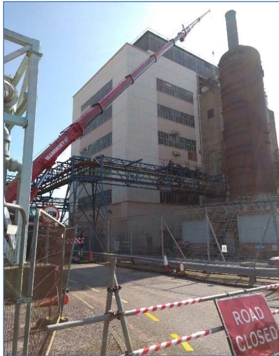
Figure 5: Removal of filter pots, Summer 2021.
