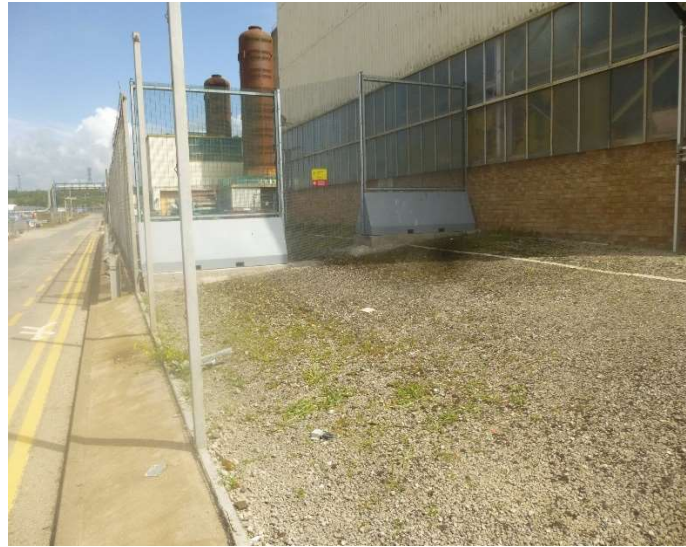
Figure 3: Reactor Compound fence removal after radiological categorisation downgraded to C1R0.
