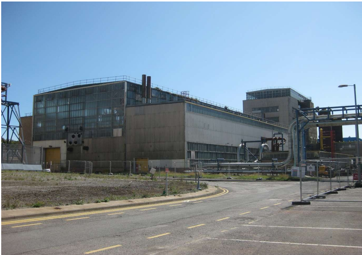
Figure 12: Turbine Hall A.
