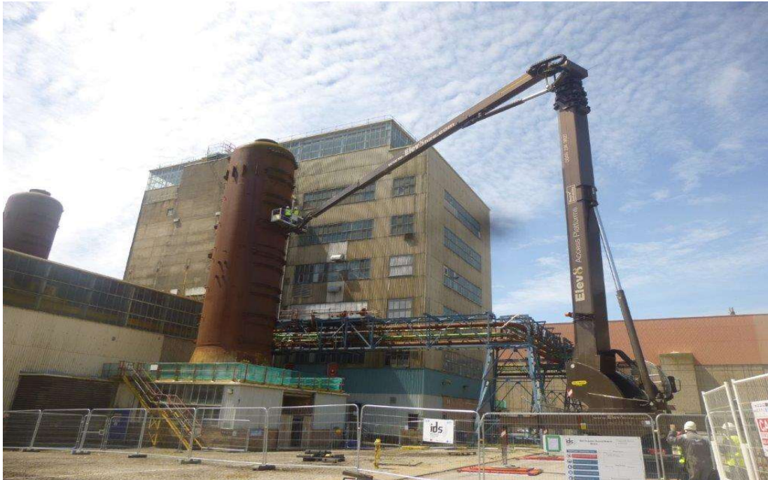
Figure 13: Work on the Reactor 1 heat exchangers.
