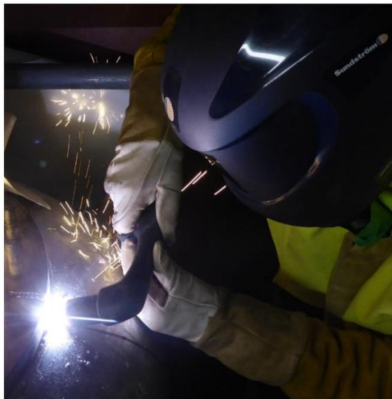
*Photograph 7: Size reducing a Caesium Removal Unit by plasma cutting*
