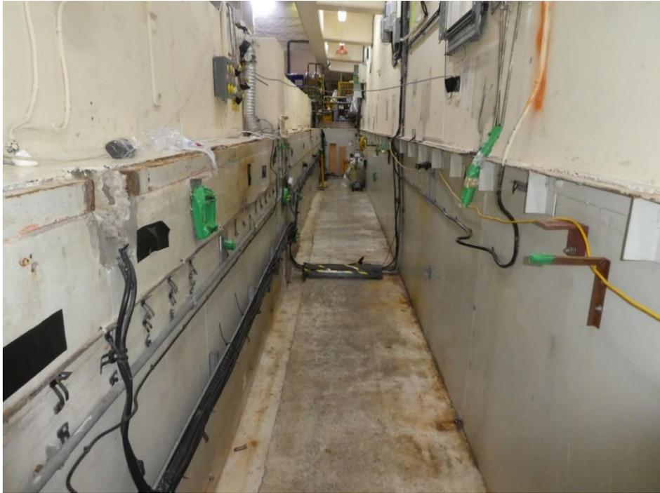
***Photograph 5: Pond's trench de-planted of contaminated pipework and ductwork***
