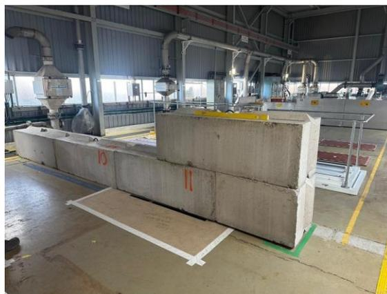
***Photograph 31: Construction of the Shield Wall to Protect Operators from Dose***
