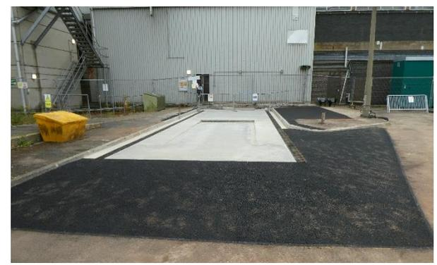
**Photographs 18 - 21: Foundation preparation for the Vacuum Fill House**
