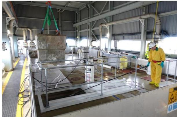
***Photograph 29: Removal of Vault Plug following installation of new Shielded 'Gamma Gates'***
