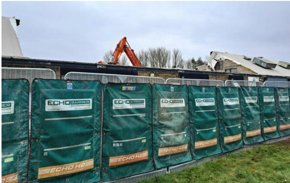
Photograph 9: Acoustic barriers used to reduce noise disturbance during the demolition of OTC
