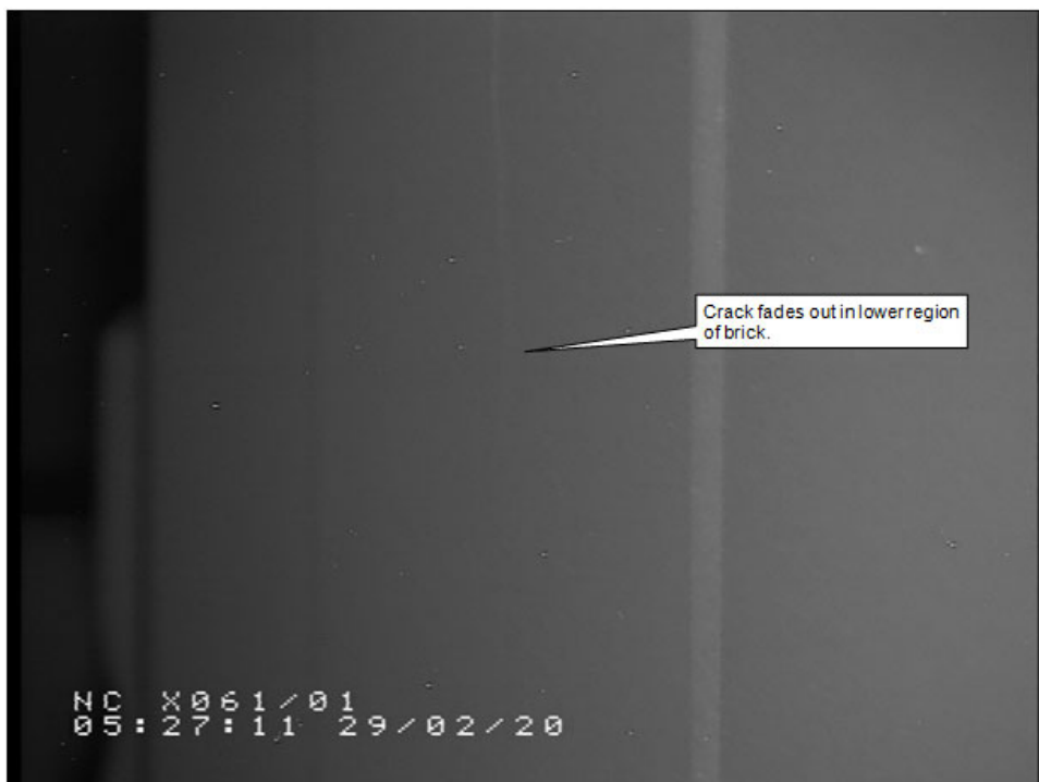
Figure 4: Cracked brick in Layer 4 of Face 15, Brick No. 2 (bottom of the brick).
