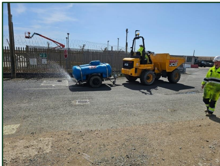
Figure 4 Use of mobile water bowser for dust suppression during the Turbine Hall infill works
