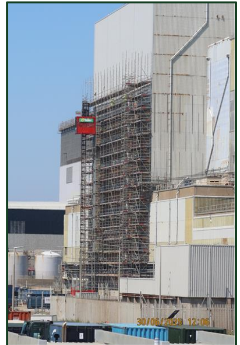
Figure 2 Reactor 2 South-side with partial completion and ongoing cladding works
