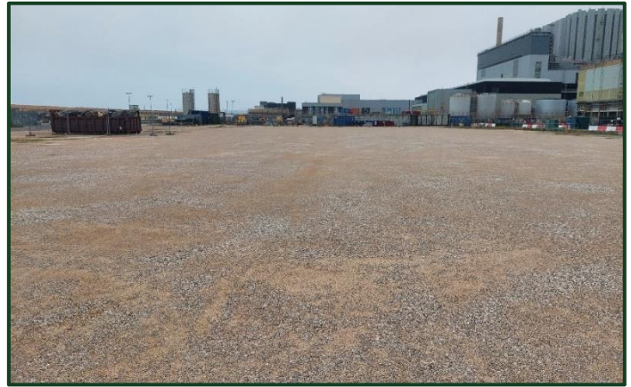
Figure 1 Completed Turbine Hall Basement Infill
