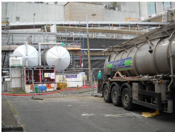
Photographs 14 and 15: The AETP Acid & Caustic Tanks draining operation, and the sludge encountered in
