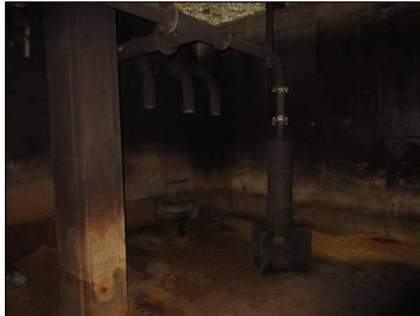
Photograph 13: The MWTP Effluent Sump A & B Internals
