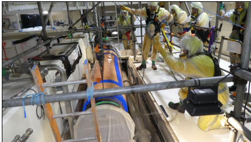
Photograph 6: Heat Exchanger being removed from trench
