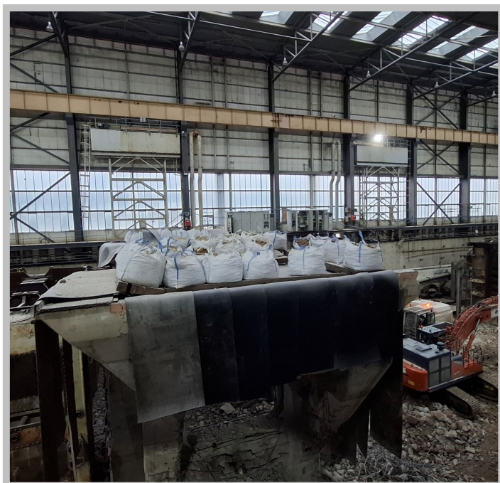
Figure 6: Explosives Positioned in Concrete Plinths
