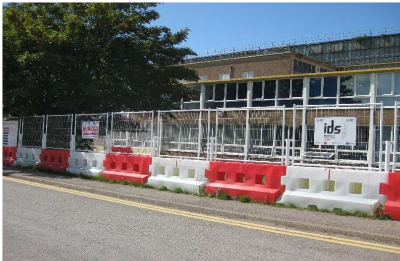
Figure 2: Redundant Administration Building now demolished.
