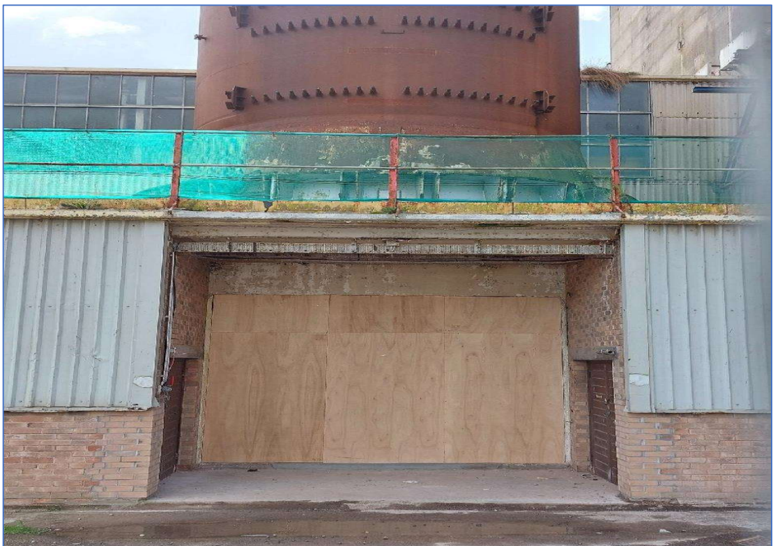
Figure 13: Weatherproofed Base of Heat Exchanger after removal of elbows & bellows.
