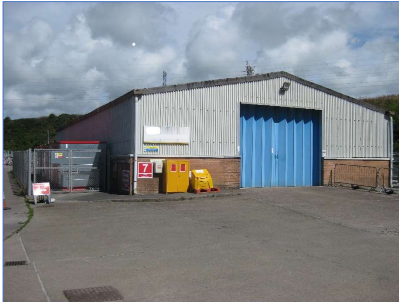
Figure 6: The Chemical Disposal Hub at Calder.
