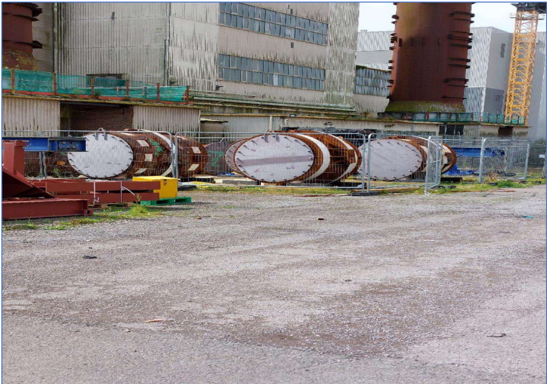
Figure 11: Removed sections of elbows & bellows from reactor 1 Heat Exchangers awaiting disposal.
