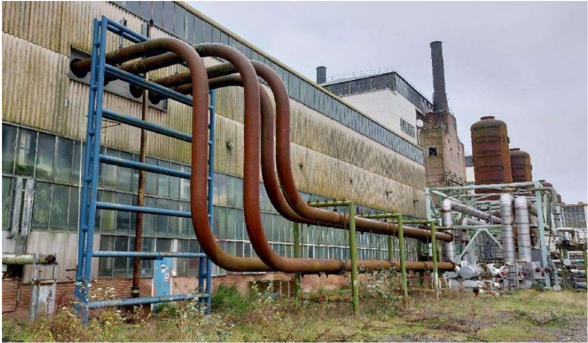
Figure 4: Turbine Hall B – West Duct Work prior to removal.
