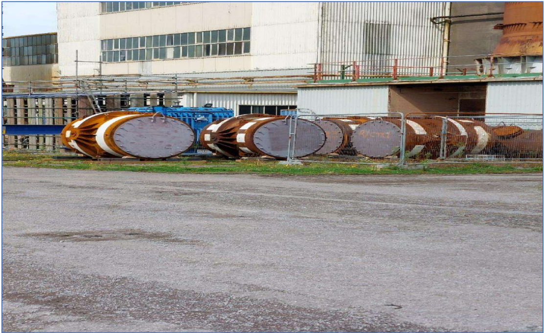
Figure 12: Removed sections of elbows & bellows from reactor 1 Heat Exchangers awaiting disposal.
