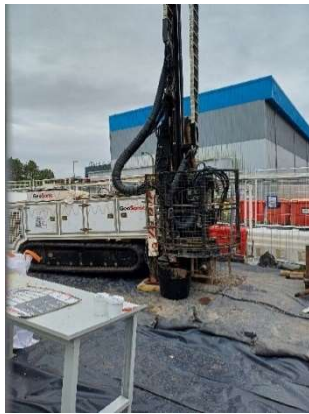
Figure 22 Hex 1 Borehole drilling
