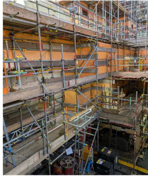
Figure 25 – TH-A Asbestos Enclosure
