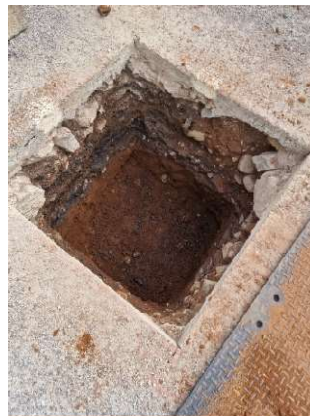
Figure 23 Hex 1 Sample test pit
