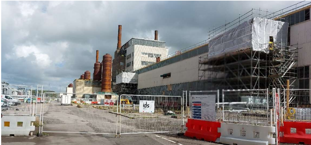
Figure 2: Showing cleared CLC Area to SIXEP side of Calder Hall Site and Turbine Hall A access towers for facilitating Asbestos clear/de-planting
