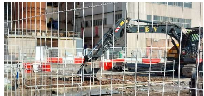
Figure 8 TH-B Water Treatment Plant Sump infill
